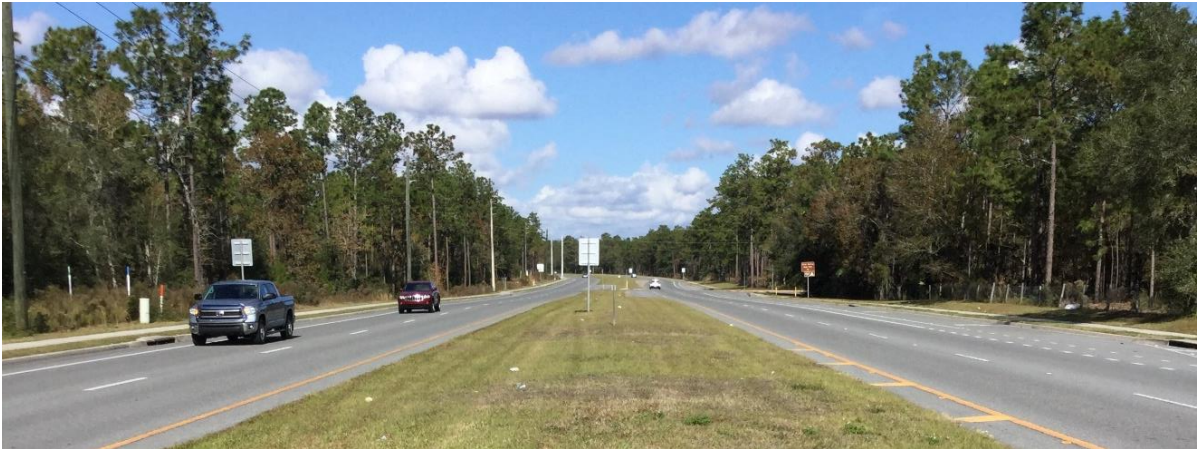
Photograph 1 – Looking north on SR 35 from the proposed crossing location
