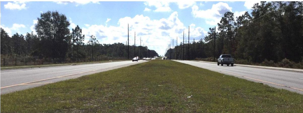
Photograph 2 – Looking south on SR 35 from the proposed crossing location
