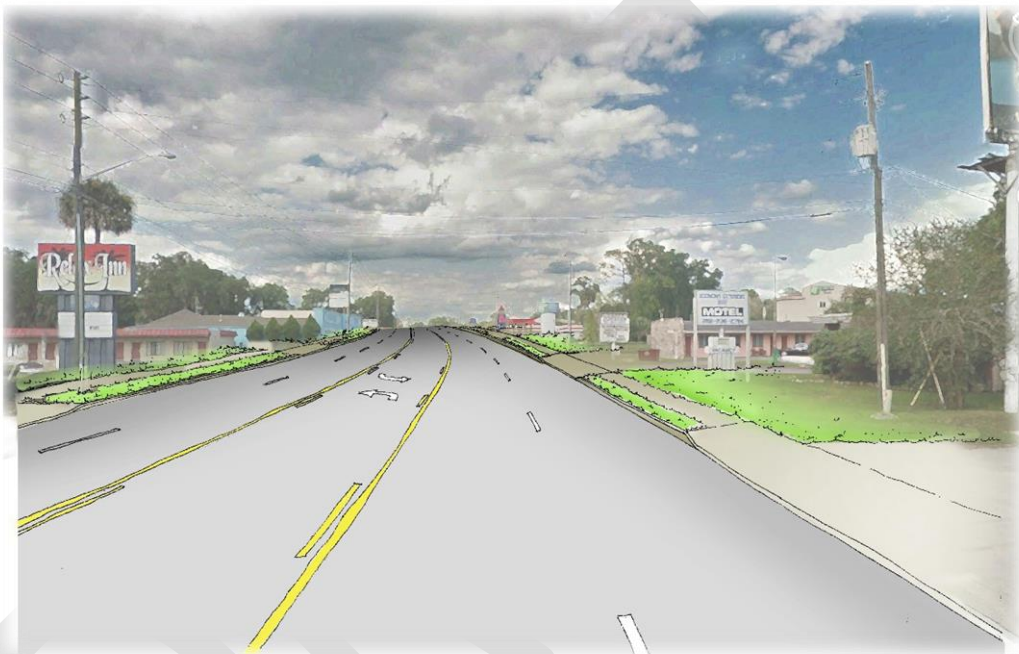
Figure 10: Perspective View – Existing Two-Way Left-Turn Lane Median
