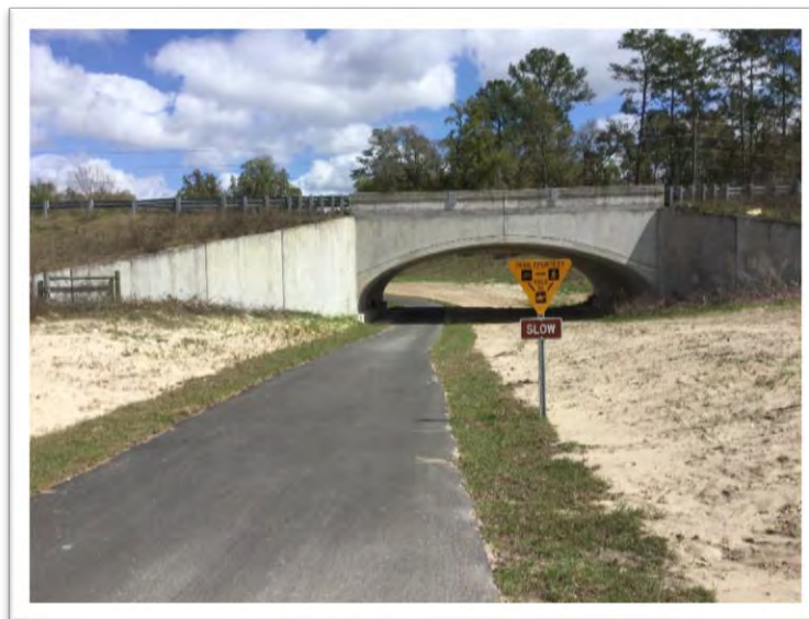
Underpass and trail etiquette signage on the Cross Florida Greenway
