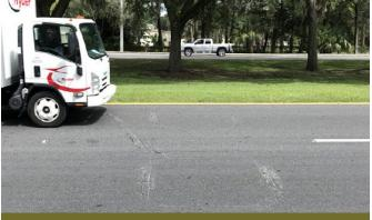
Permanent count station are sites that feature infrastructure that has been installed into the roadway surface. 'Loops' replace the use of pneumatic tubes used in temporary stations. Thesesubsurface loops are fixed and can be connected to a portable count computer or a permanent cabinet. These stations allow for basic counts, and the capability to determine vehicle class and speed.
