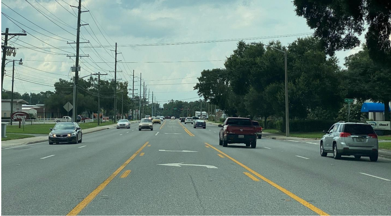
LOS C – NW 27 th Avenue, south of US 27
