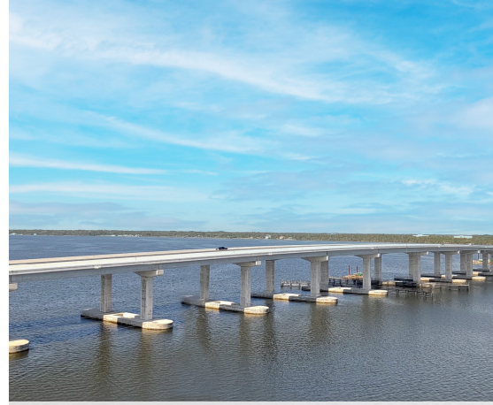
NASA Causeway Bridge, Brevard County
