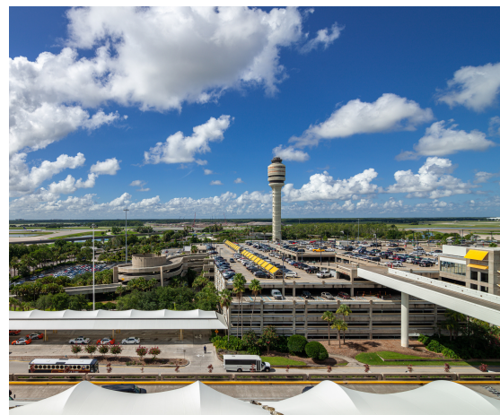
Orlando International Airport, Orange County
