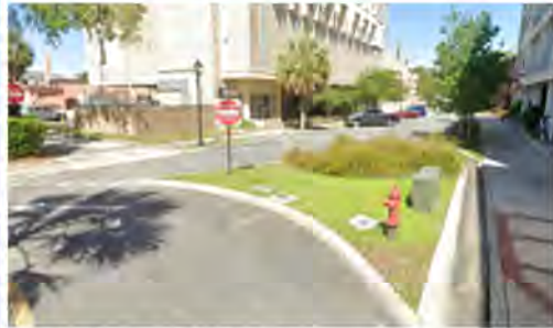
Traffic diverter in Ocala, FL
