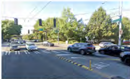
Hardened Centerline in Seattle, WA
