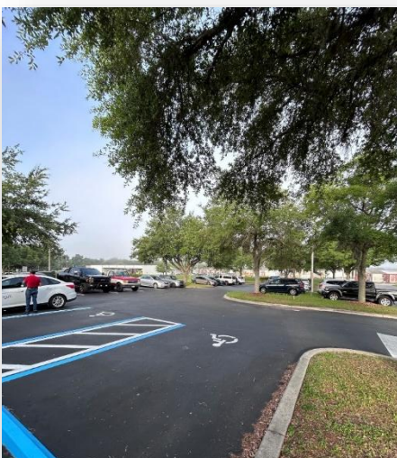
Renovated Parking Area
